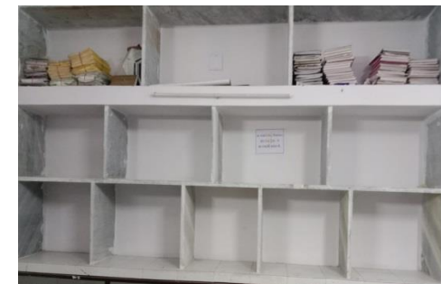
Construction of Physics Lab Rack
