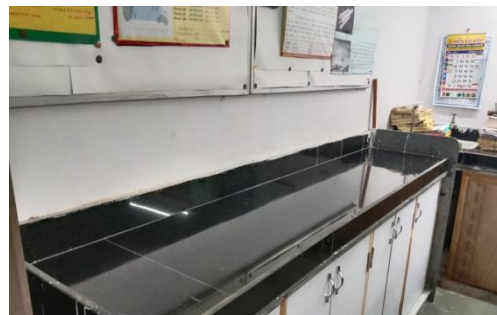
Construction of Cup-board-Physics department
