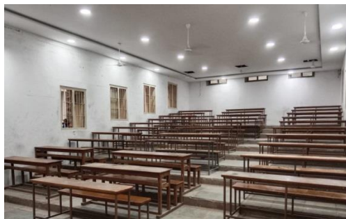
Classroom Renovation-wall painting, wall plaster, ceiling, LED strip light etc.
